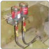
Pressure build-up to 4 bar allows remote mounting with lines up to 1 meter\*
