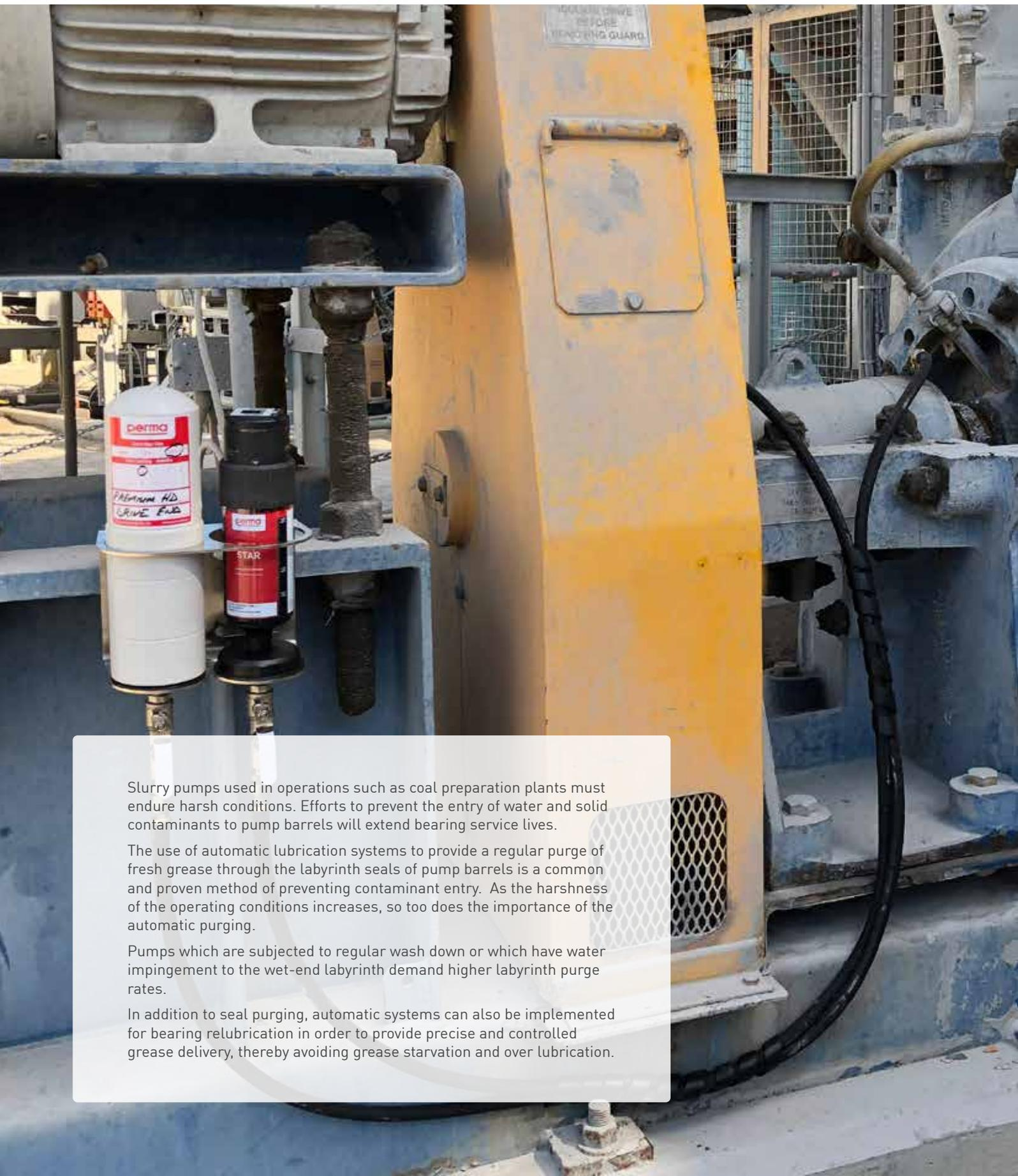
Slurry pumps used in operations such as coal preparation plants must endure harsh conditions. Efforts to prevent the entry of water and solid contaminants to pump barrels will extend bearing service lives.
