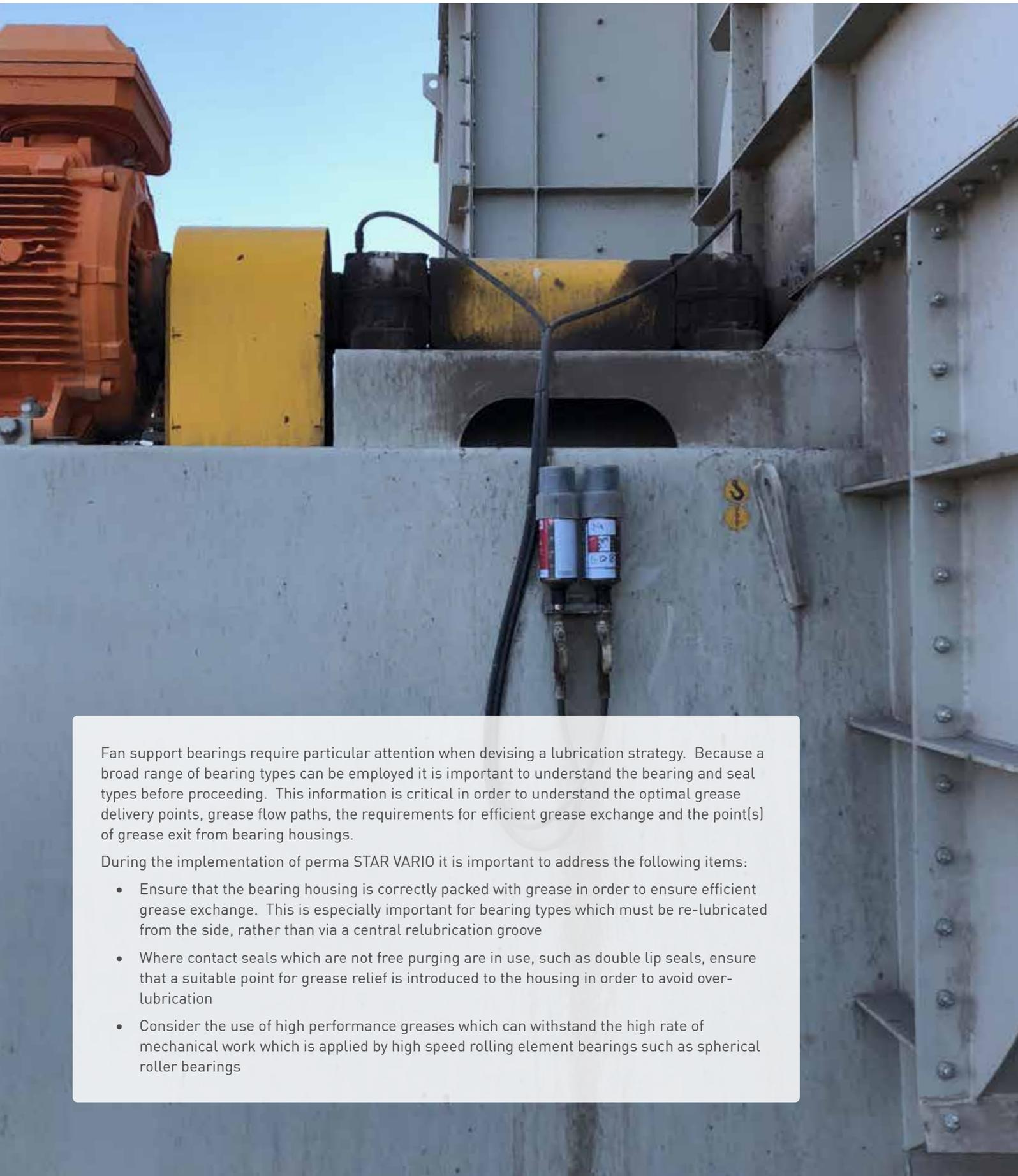
Fan support bearings require particular attention when devising a lubrication strategy. Because a broad range of bearing types can be employed it is important to understand the bearing and seal types before proceeding. This information is critical in order to understand the optimal grease delivery points, grease flow paths, the requirements for efficient grease exchange and the point(s) of grease exit from bearing housings.
