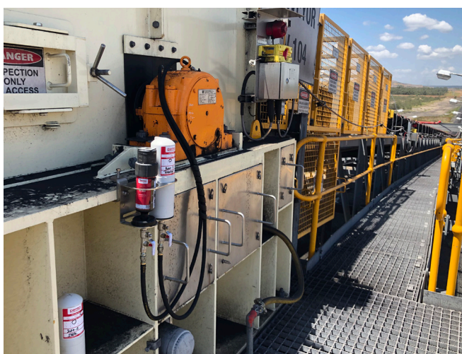
Application Conveyor pulley bearing and seal Lubricator perma STAR VARIO 250 cm³ Installation kit K230C
