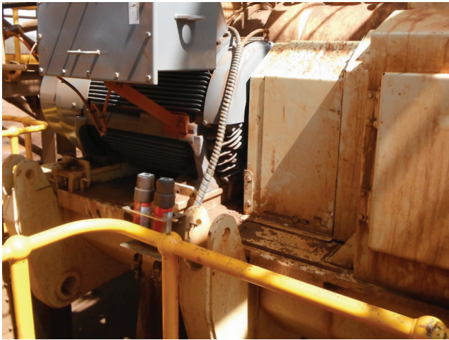
Application Electric motor Lubricator perma STAR VARIO 250 cm³ Installation kit K230C
