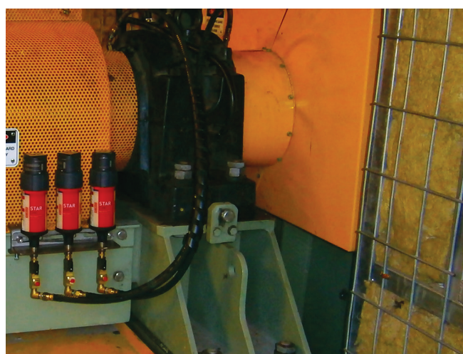
Application Fan support bearings Lubricator perma STAR VARIO 250 cm 3 Installation kit K330
